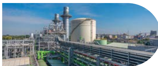
POWER GENERATION AND WATER TREATMENT
